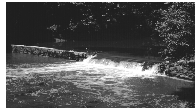
Dam on Poquessing Creek.
